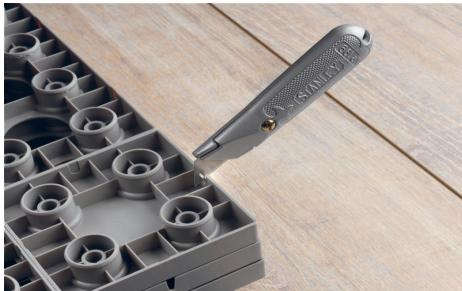
Use the openings made to determine where the screws are to be mounted, height 10mm from the floor.
