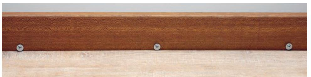
Now place the Threshold Ramp over the screw/washer.
